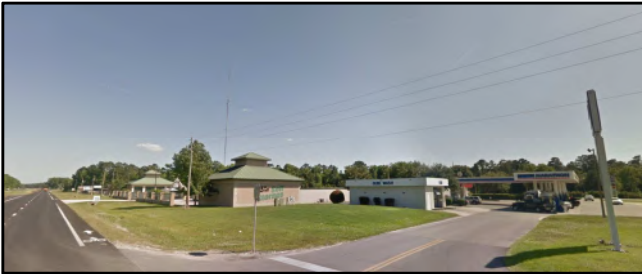
Commercial uses, Southeast of NW 43 rd Street
