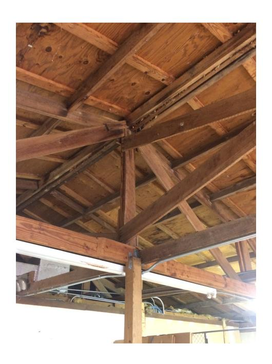
Picture 6 Column to Shore Roof Framing
