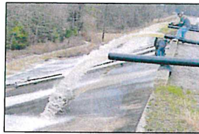
Crews work to replace drainage pipes at the Oktibbeha County Lake dam Tuesday in Starkville, Miss., as heavy rains cause water levels to rise. (RYAN PHILLIPS/STARKVILLE DAILY NEWS VIA THE ASSOCIATED PRESS)
